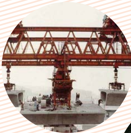
Kwun Tong Bypass First project in Hong Kong that involved segmental deck construction.
