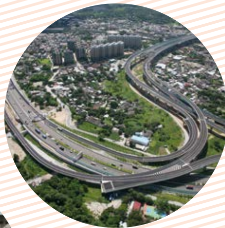
Deep Bay Link A 5.4km dual three-lane expressway comprising viaduct and bridge structures
