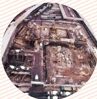
Exchange Square I & II Supervising construction of 400 large diameter bored piles in 6 months, a real race against the clock on this sleepless site! He also supervised the piling to structural topping out of Exchange Square III.
