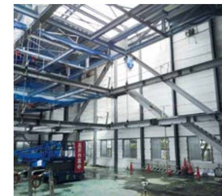
■ Centre ceiling removed, and the 2 nd and 3 rd storey frames being hung from the truss
