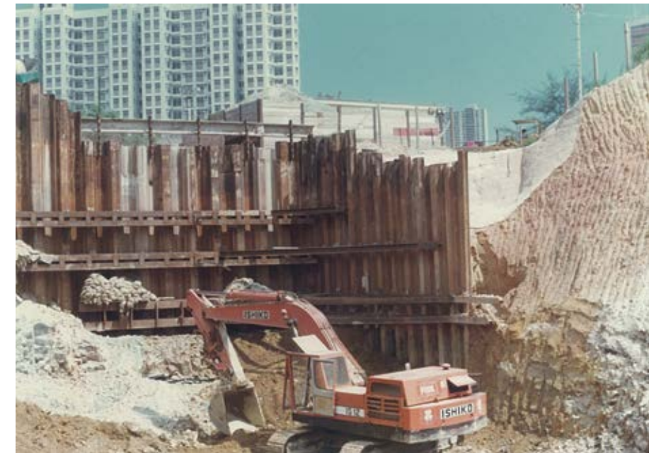
■ Timothy also designed the temporary sheetpile anchor wall for the approach tunnels
