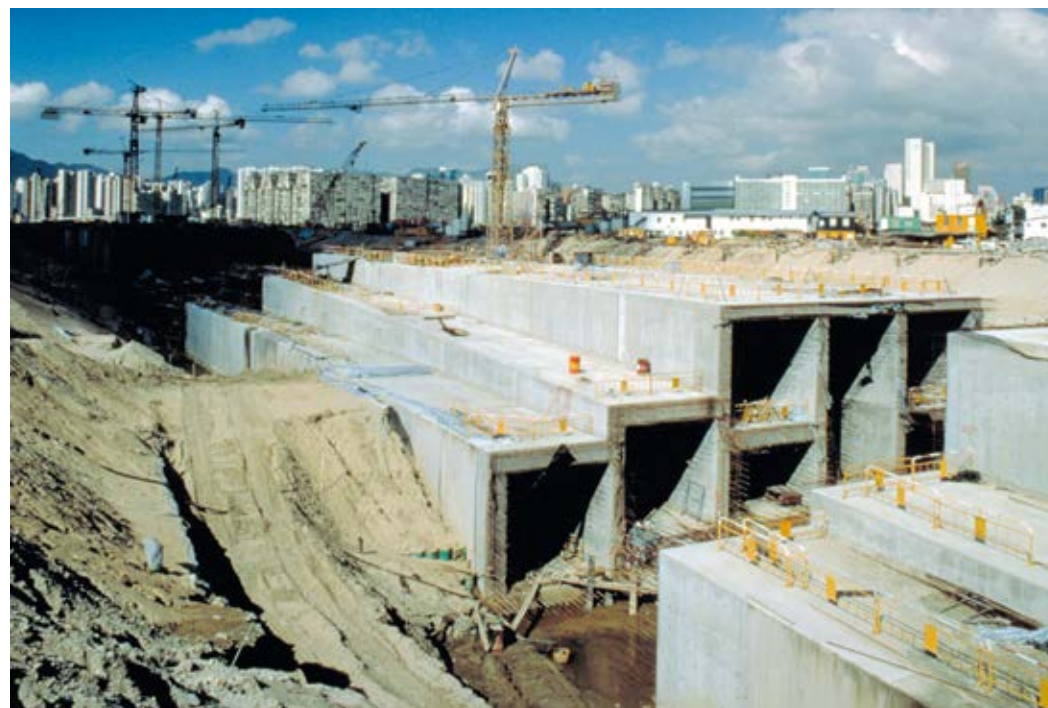
■ Cut-and-cover tunnels with 'stitching strip' gap. The temporary stitch joints allow movement of the tunnels during construction
