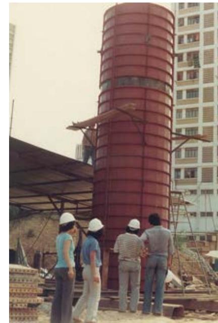
■ Timothy (third from right) at the Dragages JV site, inspecting the workmanship of a circular column formwork he designed.
